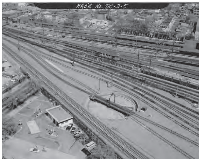
Aerial Photograph, Union Station Turntable, 1977
